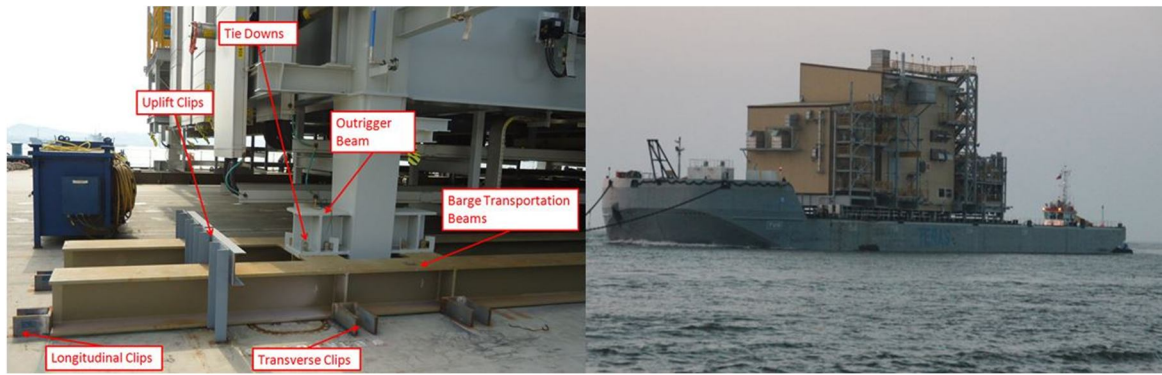
Figure 6. Structural arrangement required for a typical Ocean Transportation of Module (left) and an Image of Module on Barge (right)
